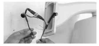
Fig. 4.2.23: Inserting cables from back
