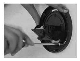
Fig. 4.2.6: Placing of camera base and fixing it
