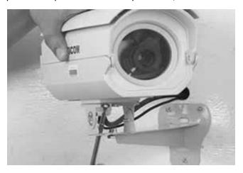
Fig. 4.2.17: Adjust the camera
