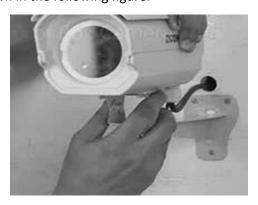
Fig. 4.2.16: Mounting and fixing the camera
